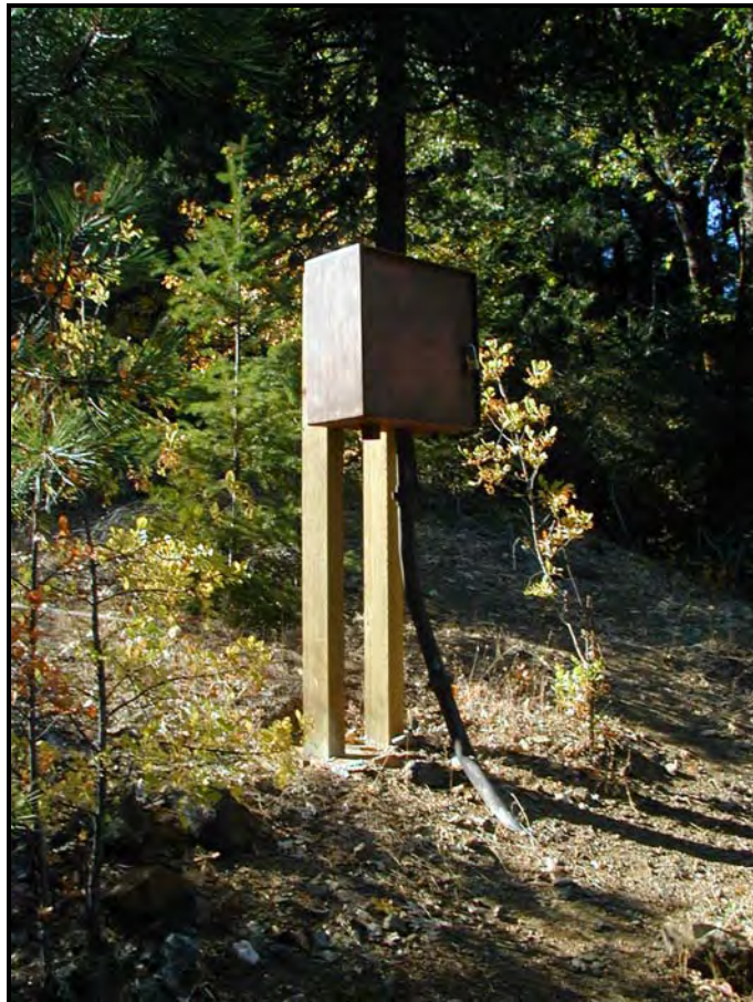
Steel gage house mounted to 4x6 posts in concrete: South Fork Trinity at Forest Glen.
