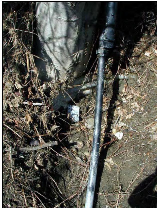
Close-up of the old USGS stilling well and inside staff plate for the Hayfork Creek near Hyampom Gage.
