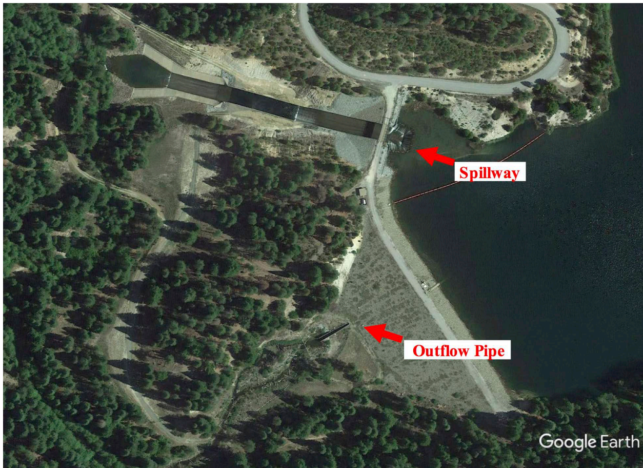
Figure 14. Buckhorn Dam, 28 May 2016. Reservoir elevation at overflow is 2803.0 ft ASL. Total dam height is 92 ft.
