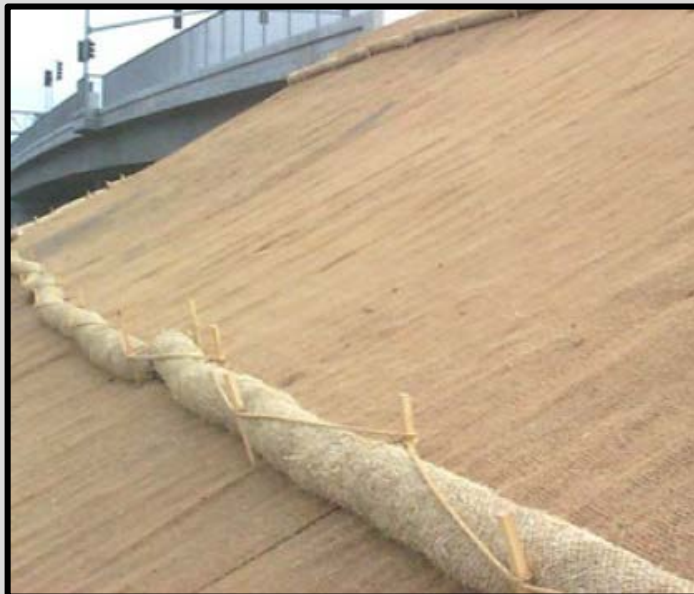
Figure 7- Typical Fiber Roll Installation (Caltrans 2017).
