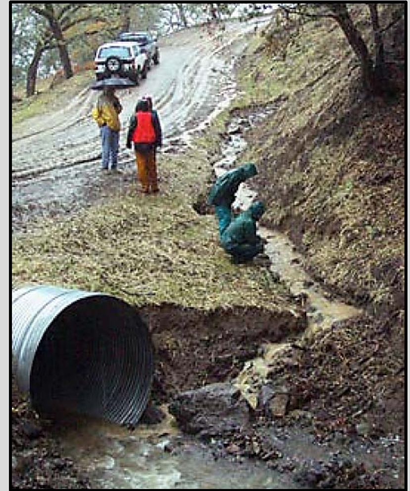
Figure 19- A Hydrologically Connected Road and Stream Channel (Weaver et. al 2015).
