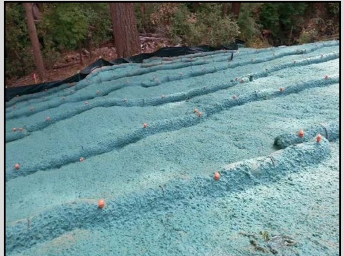
Figure 17- An Example of Hydroseeding (Caltrans 2017).
