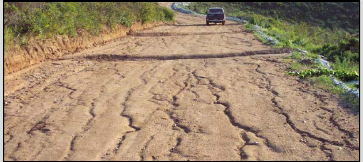
Figure 20- Rills Forming on a Natively Surfaced Road (Weaver et. Al 2015).
