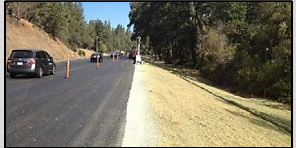
Figure 25- An Example of Mulch Applied to a Disturbed Area (Caltrans 2017).
