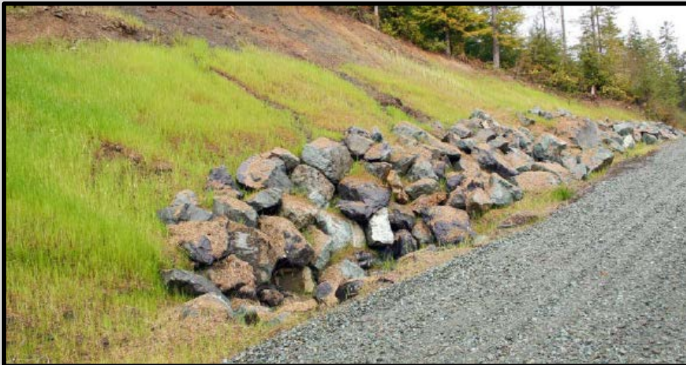
Figure 13- Rip Rap Placement for Slope Stability (Weaver et. Al 2015).
