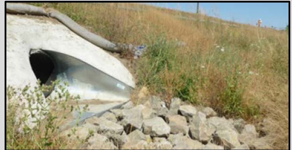
Figure 14- A Culvert with Velocity Dissipaters In Place (Caltrans 2017).
