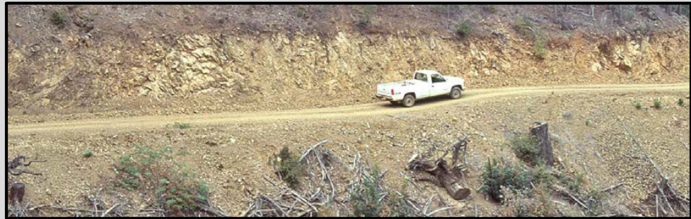
Figure 9- A Rolling Dip Installed on a Rural Access Road (Weaver et. al 2015).
