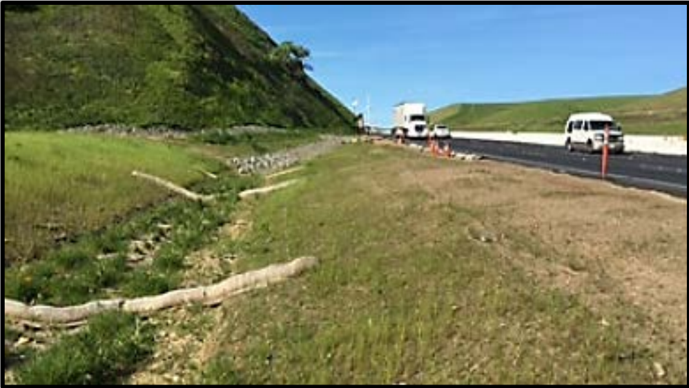
Figure 15- A Ditch with Fiber Roll Check Dams (Caltrans 2017).
