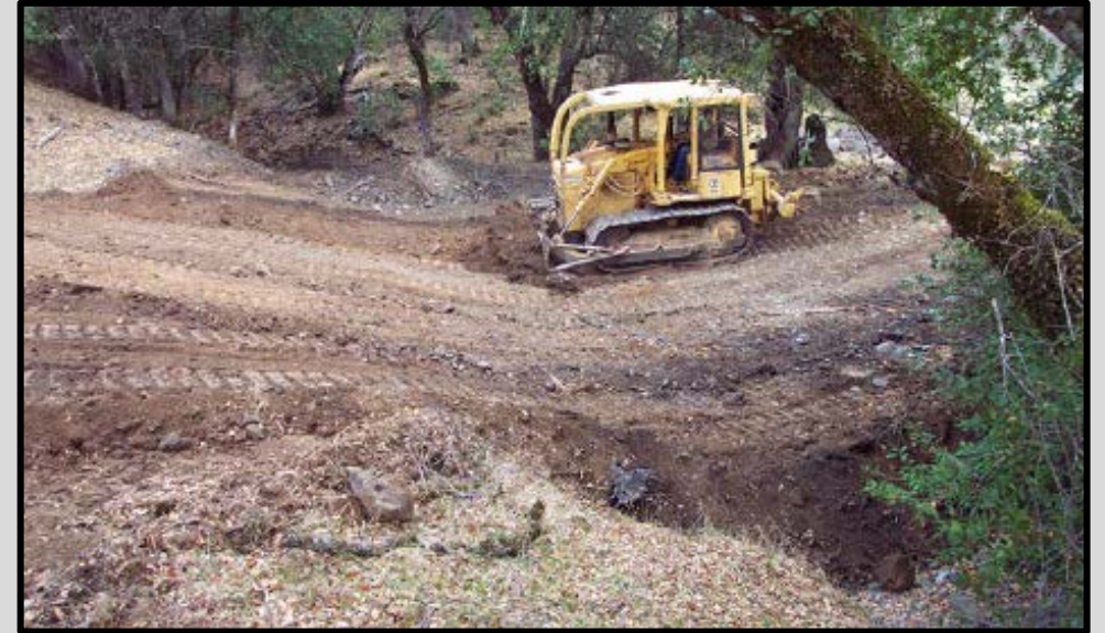
Figure 6- An Image of Instream Work in progress (Weaver et. al 2015).
