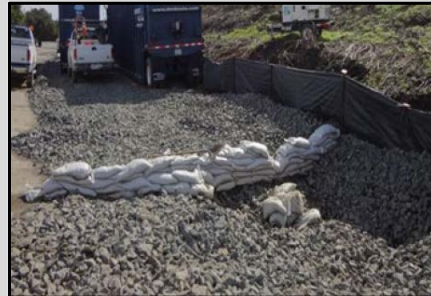
Figure 8- Typical Gravel Bag Installation (Caltrans 2017).
