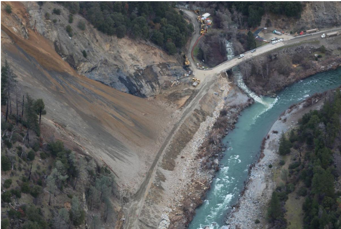
Figure 4.81 Big French Creek slide, occurred December 9, 2016. Big French Creek is the tributary entering the Trinity River under the bridge. (Photo credit – Caltrans)
