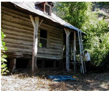
Historical Limekiln Cabin Improvements
