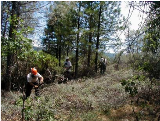
Shaded Fuel Break Construction
