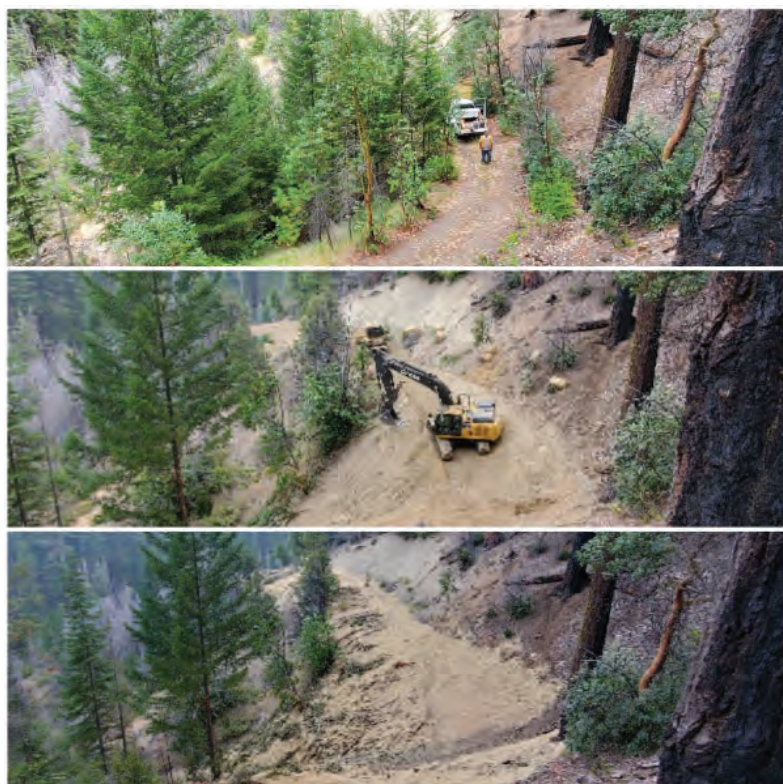
Before, during, and after shots of road decommissioning
