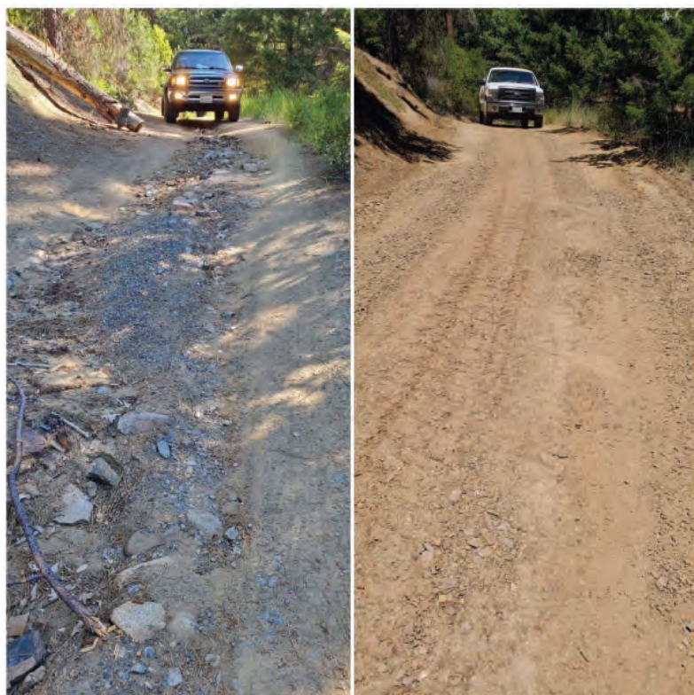
Before and after road improvements
