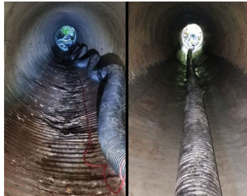
Photo 2: Before and after of culvert repair on 33N41 spur A
