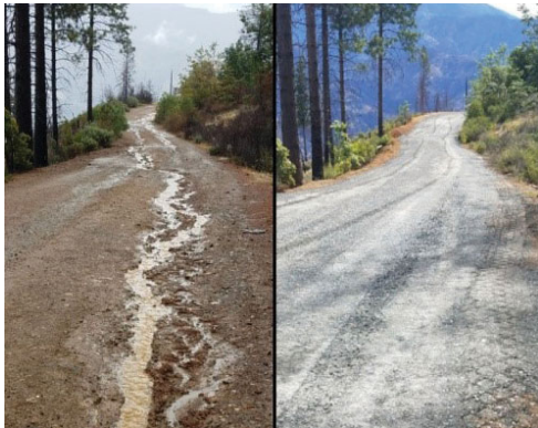
Photo 1: Before and after of road rock surfacing on Hocker Meadow Road
