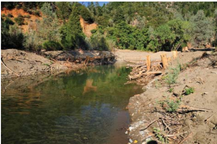
Wheel Gulch rehabilitation site after construction in 2011.
