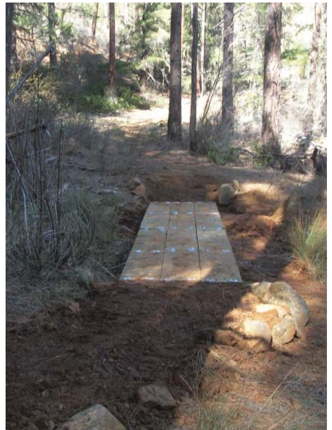
New foot bridge along Garden Gulch Spur Trail.
