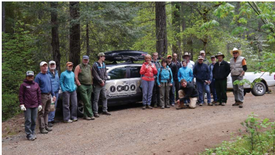
Volunteers ready to get started on the re-routing of “Misery Hill” on the Jackass Ridge Trail.
