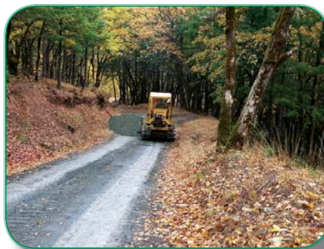
Grading on Upper Democrat Gulch Rd.
