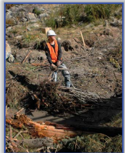
Student trainee hauling willow bundle used to create habitat for fish and other aquatic species.
