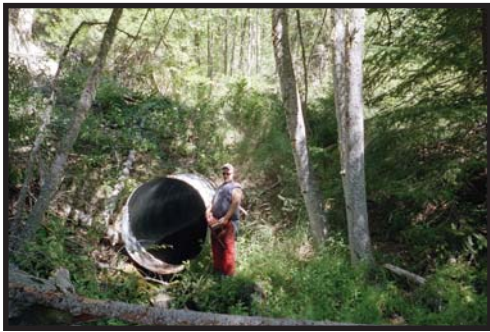
Smoky Basin, 29N11A Milemarker 0.32, 500 cubic yards excavated from stream crossing
