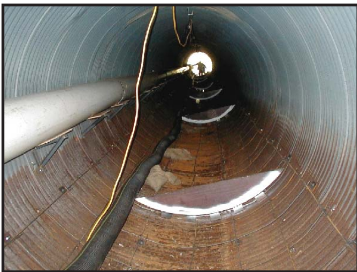
Diversion pipe, rebar, and baffles inside culvert.
