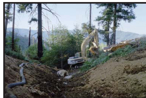
Upper South Fork Basin, 28N40 Milemarker 2.74, 1200 cubic yards excavated from stream crossing
