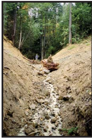
Hidden Valley Basin, 1N24A Milemarker 0.14, 2000 cubic yards excavated from stream crossing
