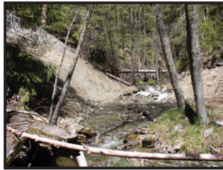
Smoky Basin, 29N11A Milemarker 0.32, 500 cubic yards excavated from stream crossing
